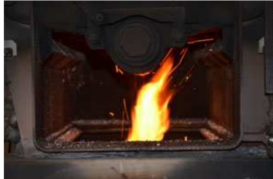
Fig. 14 Improper shape of the flame
